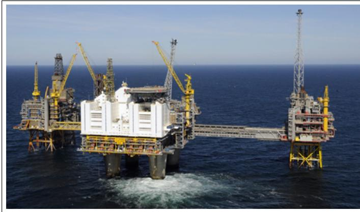
**Figure 4.3:** Concrete based and steel jacket platforms in the Oseberg field in the North Sea. *Source: Statoil*
