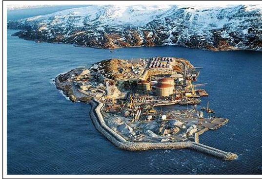
**Figure 9.10:** Icelandic type berm breakwater protecting Melkøya terminal, Norway.
