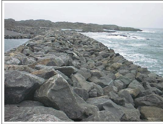
**Figure 9.9:** The Sirevåg berm breakwater after the storm in January 2002. *Source: P. Bruun, 2006*
