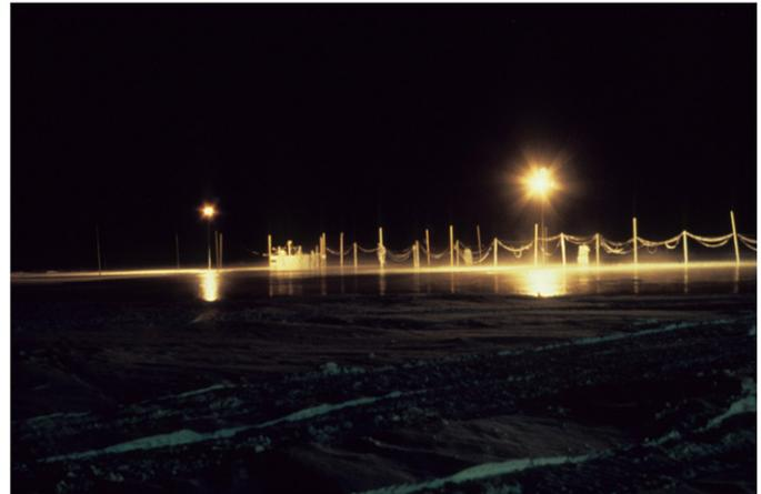
Fig. 30. Flooding an ice platform.
