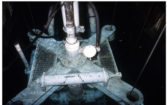
Fig. 36. Lowering the wellhead.
