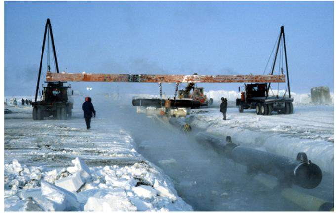
Fig. 35. Lowering pipe through the ice.
