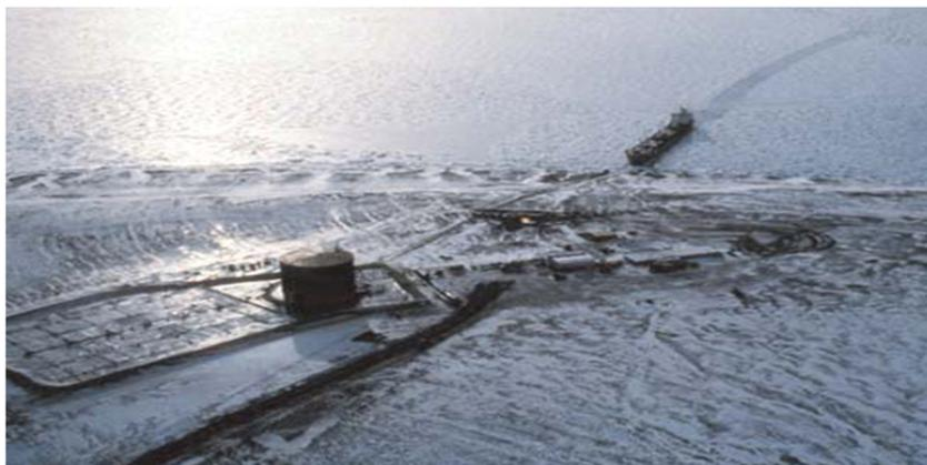
Fig. 39. Ship loading at Bent Horn from storage tank.
