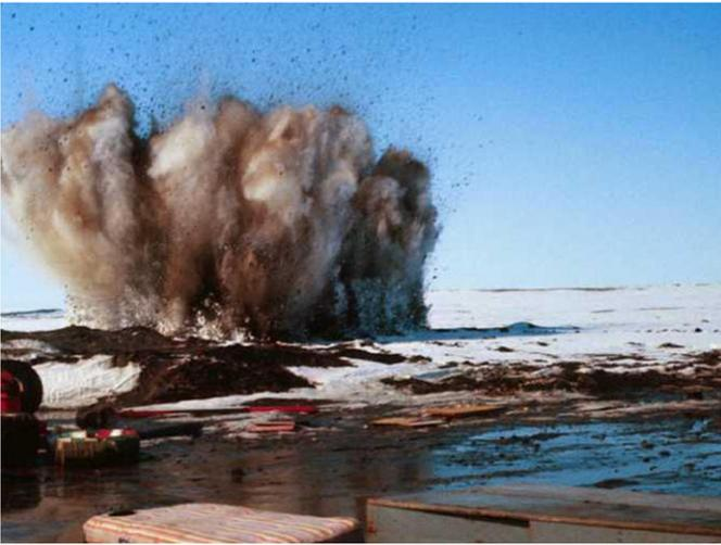
Fig. 19. Blasting a hole in the permafrost.
